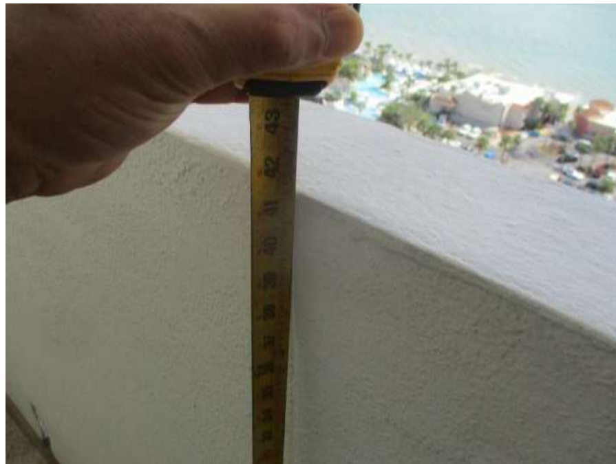
Photo #22 – Typical Guard Wall Height
