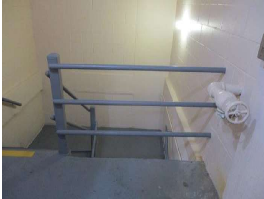
Photo #25 – Typical Stair Tower Railing at Landing and Stairs
