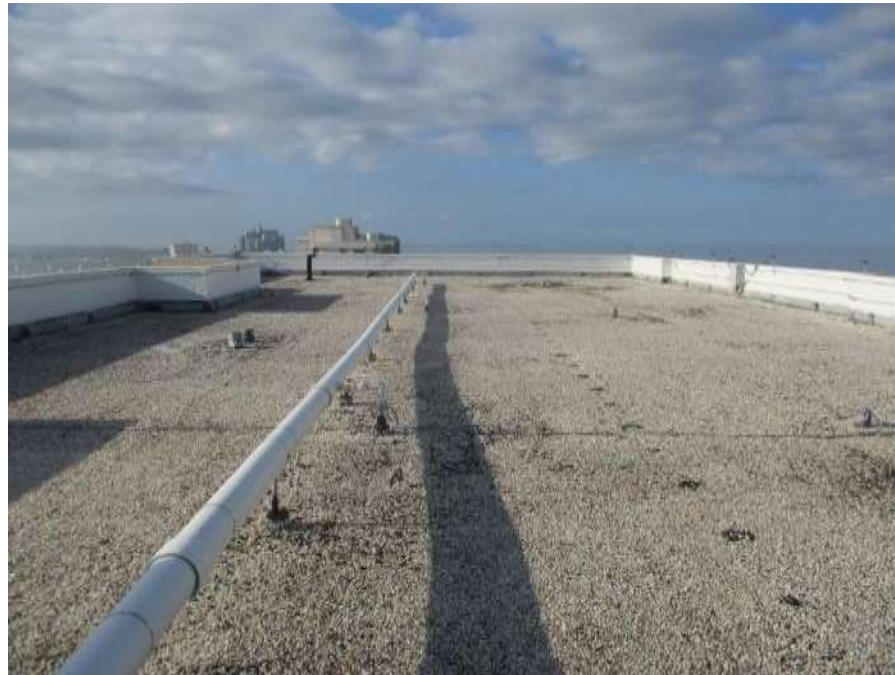
Photo #3 – Overview of Roof
