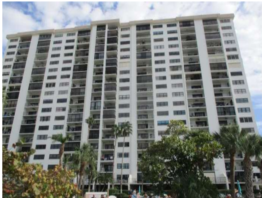
Photo #2 – West Elevation of Building
