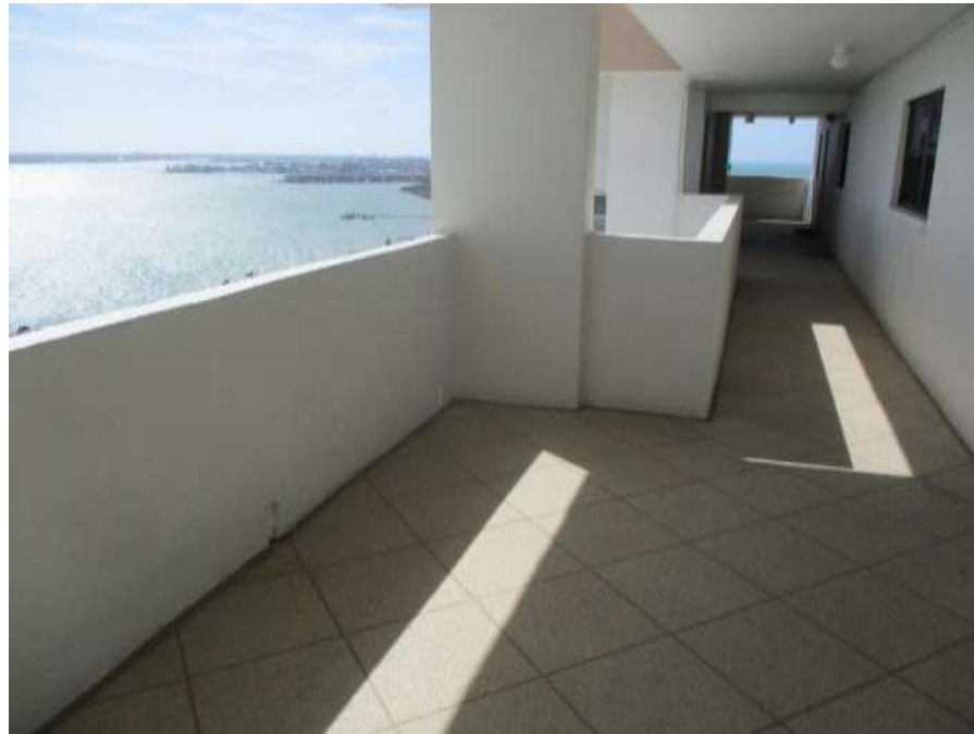
Photo #21 – Typical Elevated Walkway and Guard Wall System
