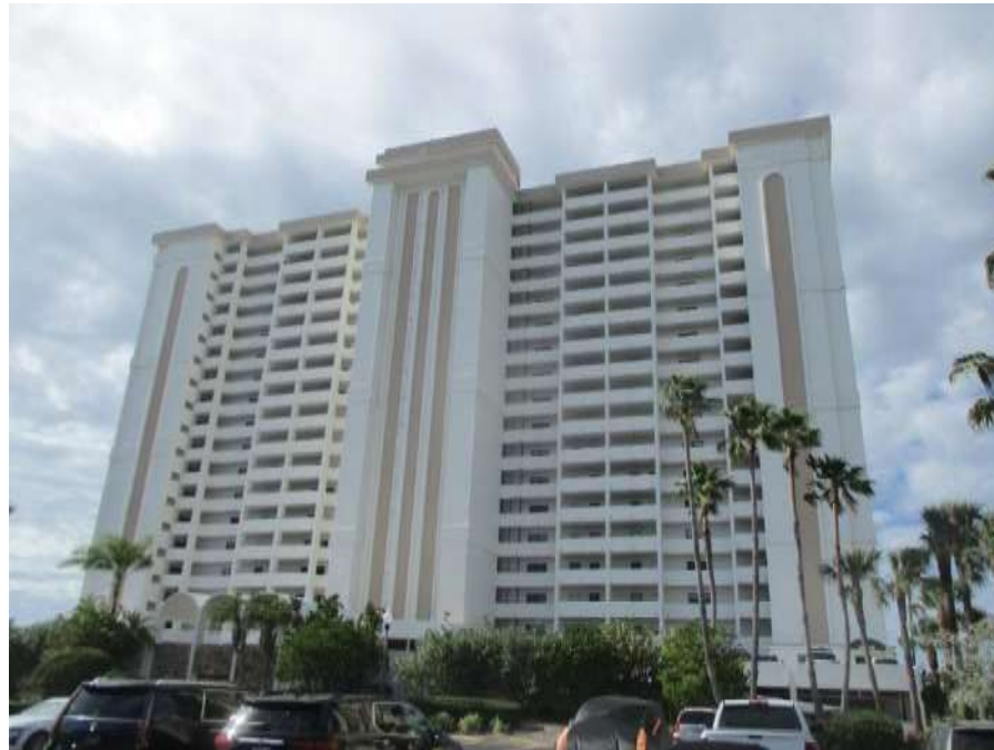
Photo #1 – East Elevation on Building
