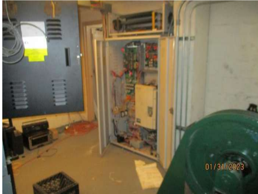
Photo #9 – In Progress Elevator Equipment Replacement
