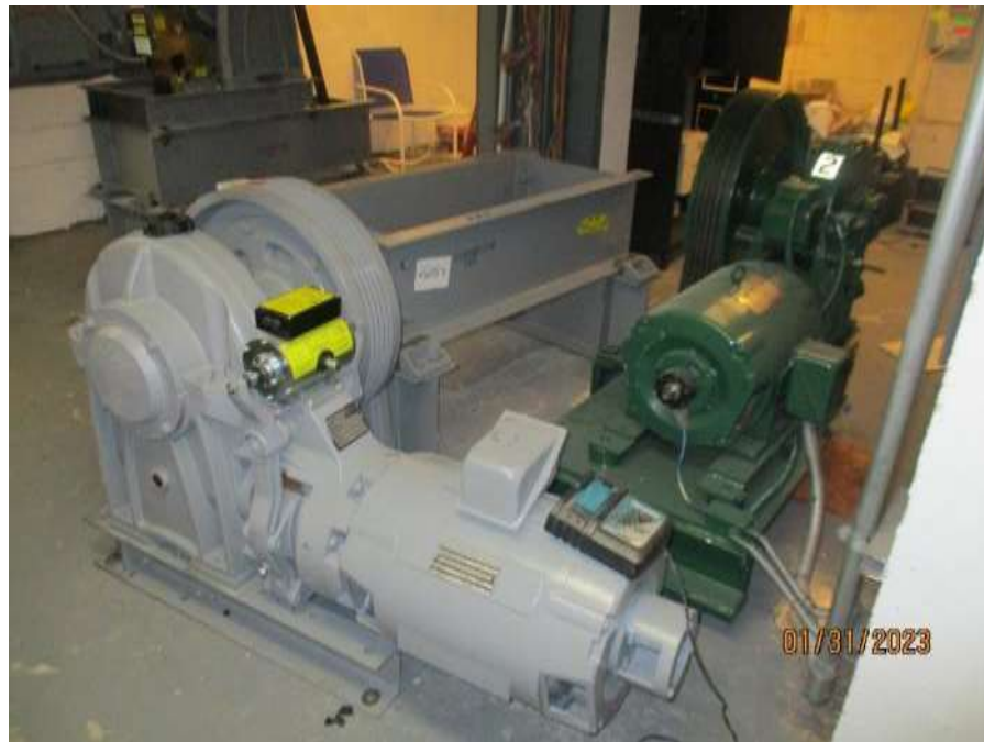
Photo #8 – In Progress Elevator Equipment Replacement
