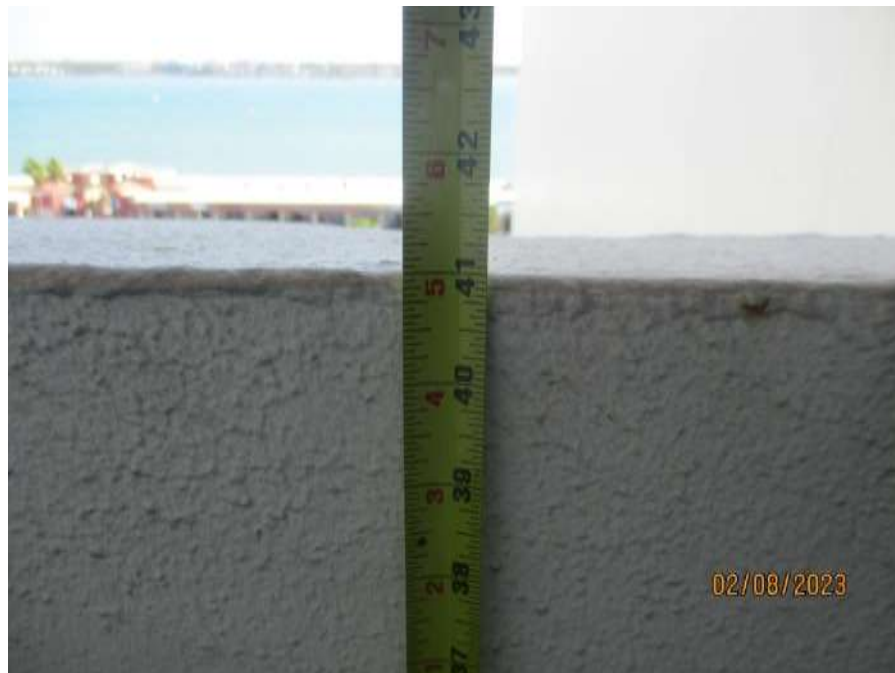
Typical Walkway Guard Wall Height = +/- 41"
