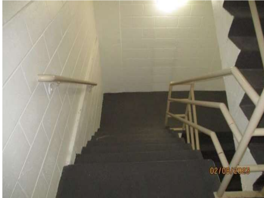
Typical Interior Stair Tower Railings
