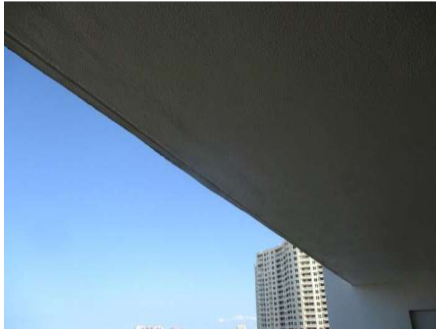
Sapling Concrete at Slab Edge
