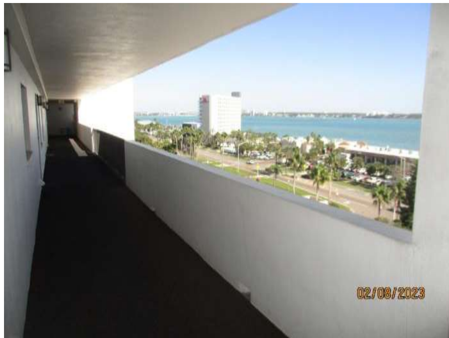
Typical Exterior Walkway
