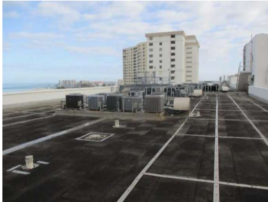
Overview of Inverted Roofing Membrane System
