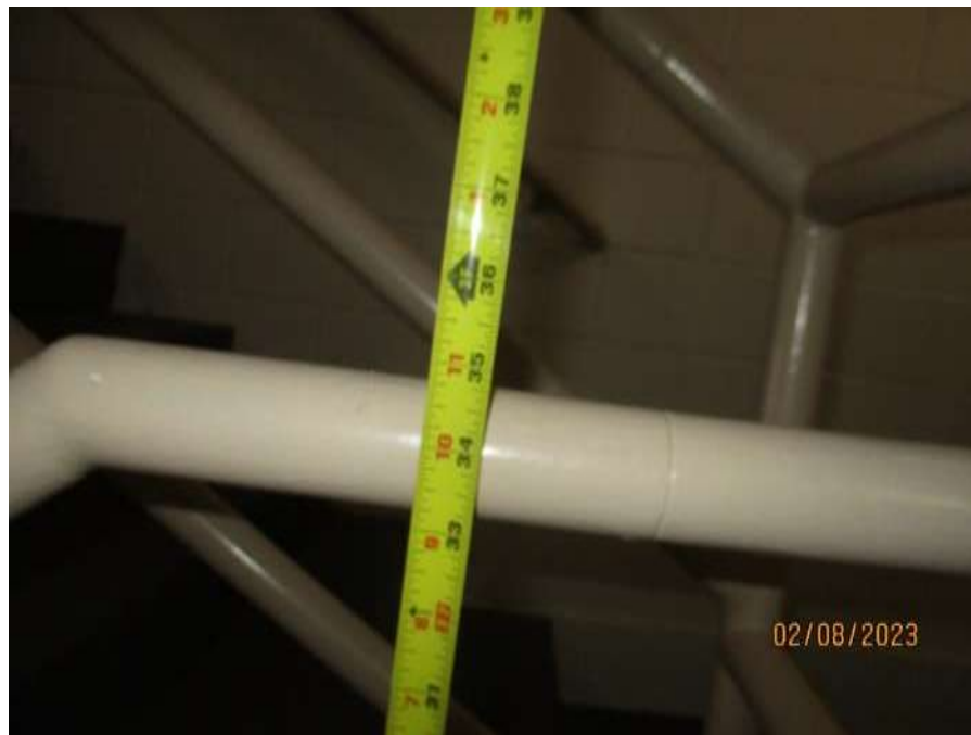
Typical Stair Tower Railing Height = +/- 35"
