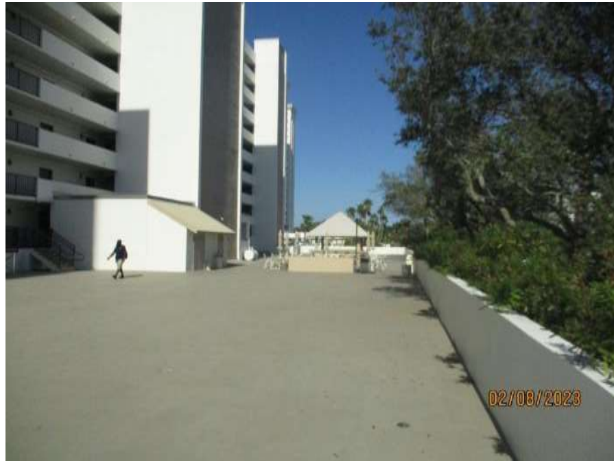
Elevated Terrace Deck at 2 nd Floor
