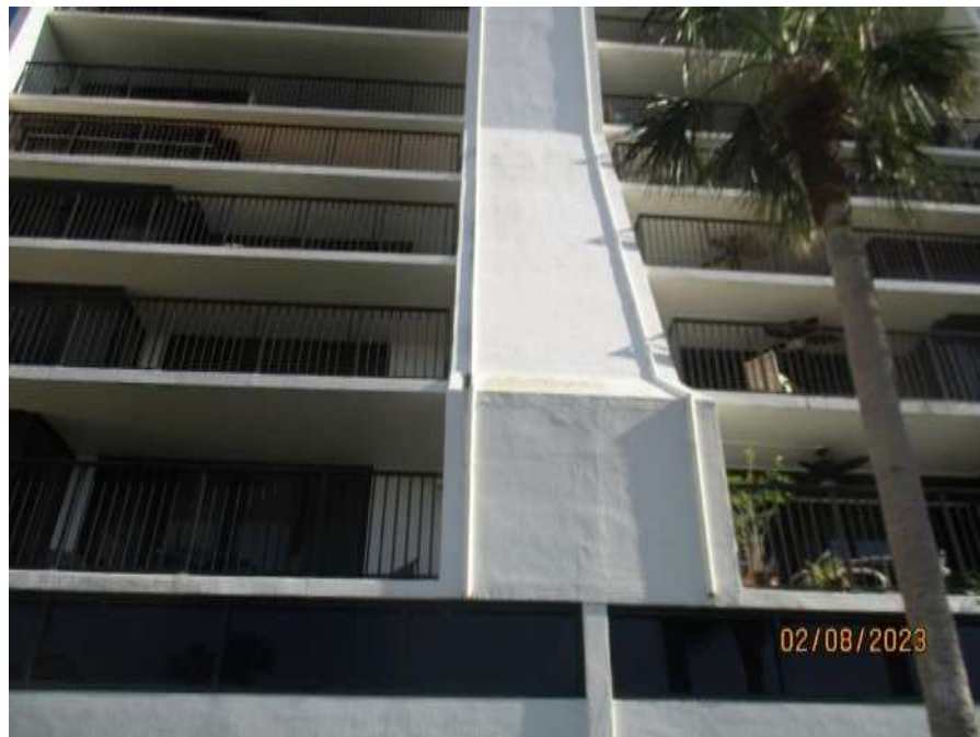
Typical Apparent Staining and Potential Water Intrusion Indicators at Sloped Roof
