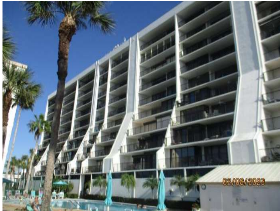
Rear Elevation of Building
